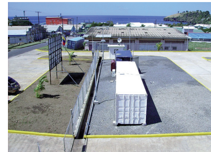
View of the entrance to the plant including guard house, 20' service container with backup power generator and 40' office container (white container)
