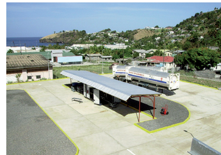
View of the filling container and the 40' ISO storage tanks
