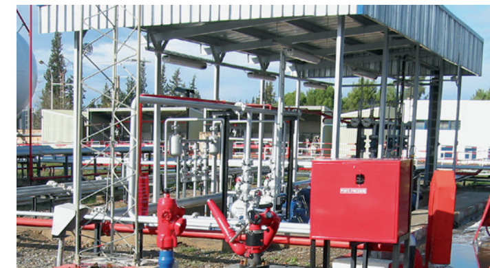
The new pump platform with two LP gas pumps with dry-running protection
