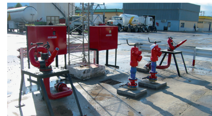
The new fire water installation including hydrants, hose cabinets and fire monitors
